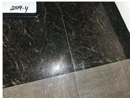
2109-4 12"x12" Floor Tile/Adhesive Typical Interior
