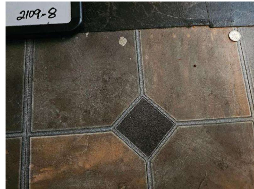
2109-8 12"x12" Floor Tile/Adhesive Typical Interior
