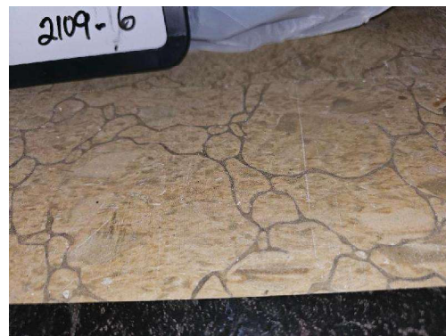
2109-6 12"x12" Floor Tile (3% Chrysotile) Typical Interior (Appx 200 sq ft)
