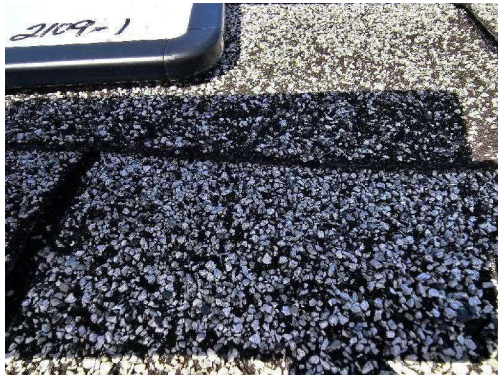
2109-1 Asphalt Shingle Typical Exterior Roof
