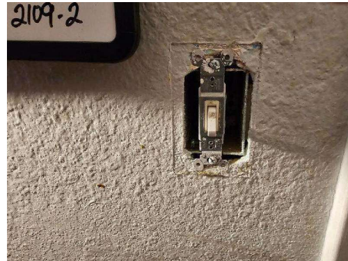
2109-2 Drywall/Joint Compound Typical Interior
