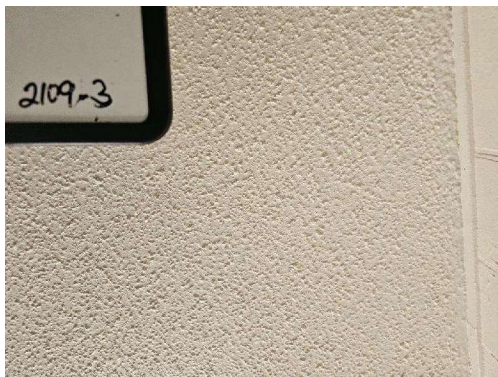
2109-3 Surfacing Material (3% Chrysotile) Typical Interior
