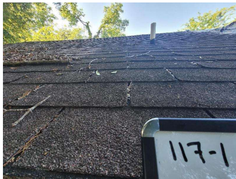
117-1 Asphalt Shingle/Tar Typical Exterior Roof
