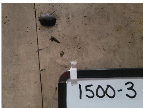
1500-3 12"x12" Floor Tile/Tan (2% Chrysotile) Mastic/Black (4% Chrysotile) Typical Interior (Bottom Layer) Appx. 650 sf
