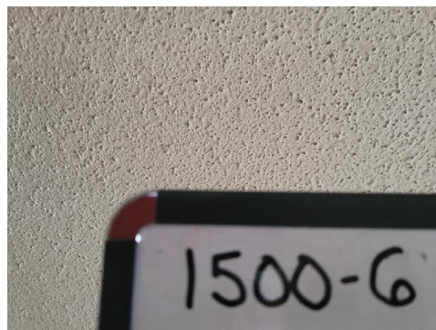
1500-6 Popcorn Texture/White (2% Chrysotile) Typical Interior Ceilings/Appx. 800 sf
