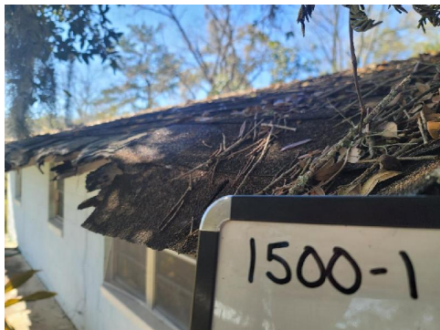
1500-1 Asphalt Shingle/Tar Typical Exterior Roof
