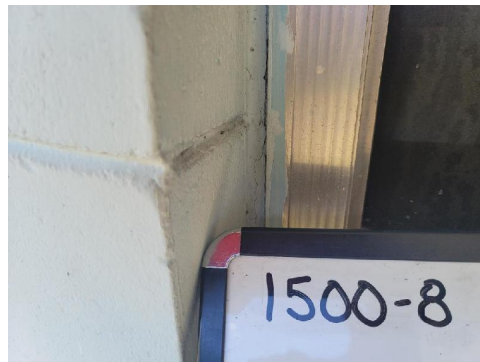
1500-8 Glazing/Off-White (2% Chrysotile) Typical Exterior Windows
