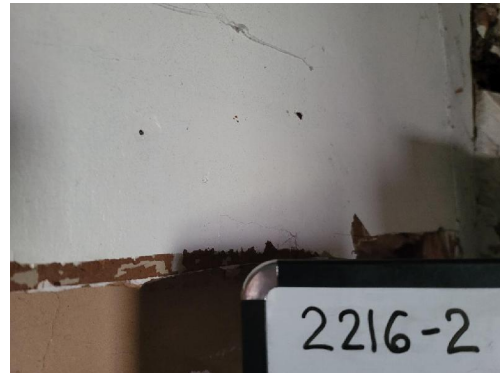
2216-2 Drywall Typical Interior Walls
