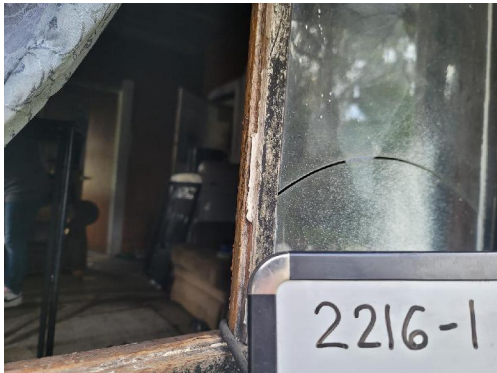
2216-1 Caulk Typical Exterior Windows
