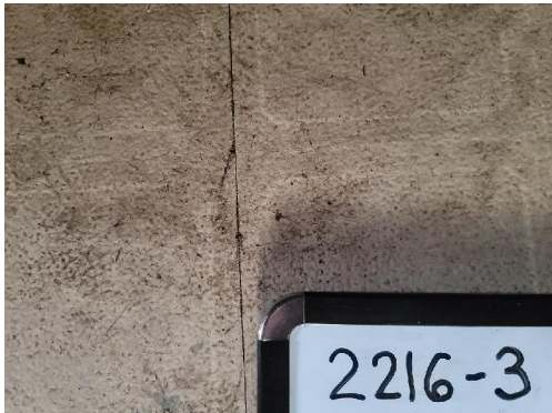
2216-3 12"x12" Floor Tile/Mastic Interior Living Room
