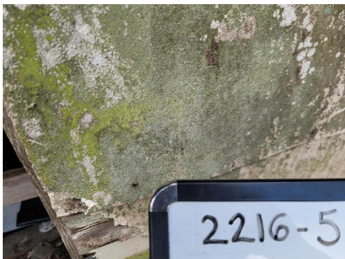
2216-5 Siding Exterior Front Porch Wall
