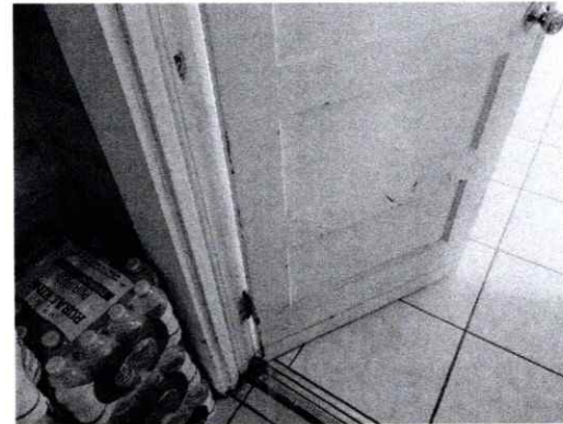
Laundry Room(004) A-Wall, Left Wood Door and Jamb Lead-Positive, Deteriorated
