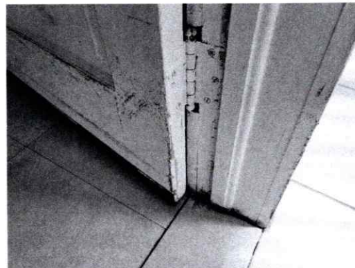
Front Room(001) C-Wall, Center Wood Door and Jamb Lead-Positive, Deteriorated
