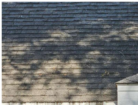
2330-3 Asphalt Shingle/Tar Typical Exterior Roof
