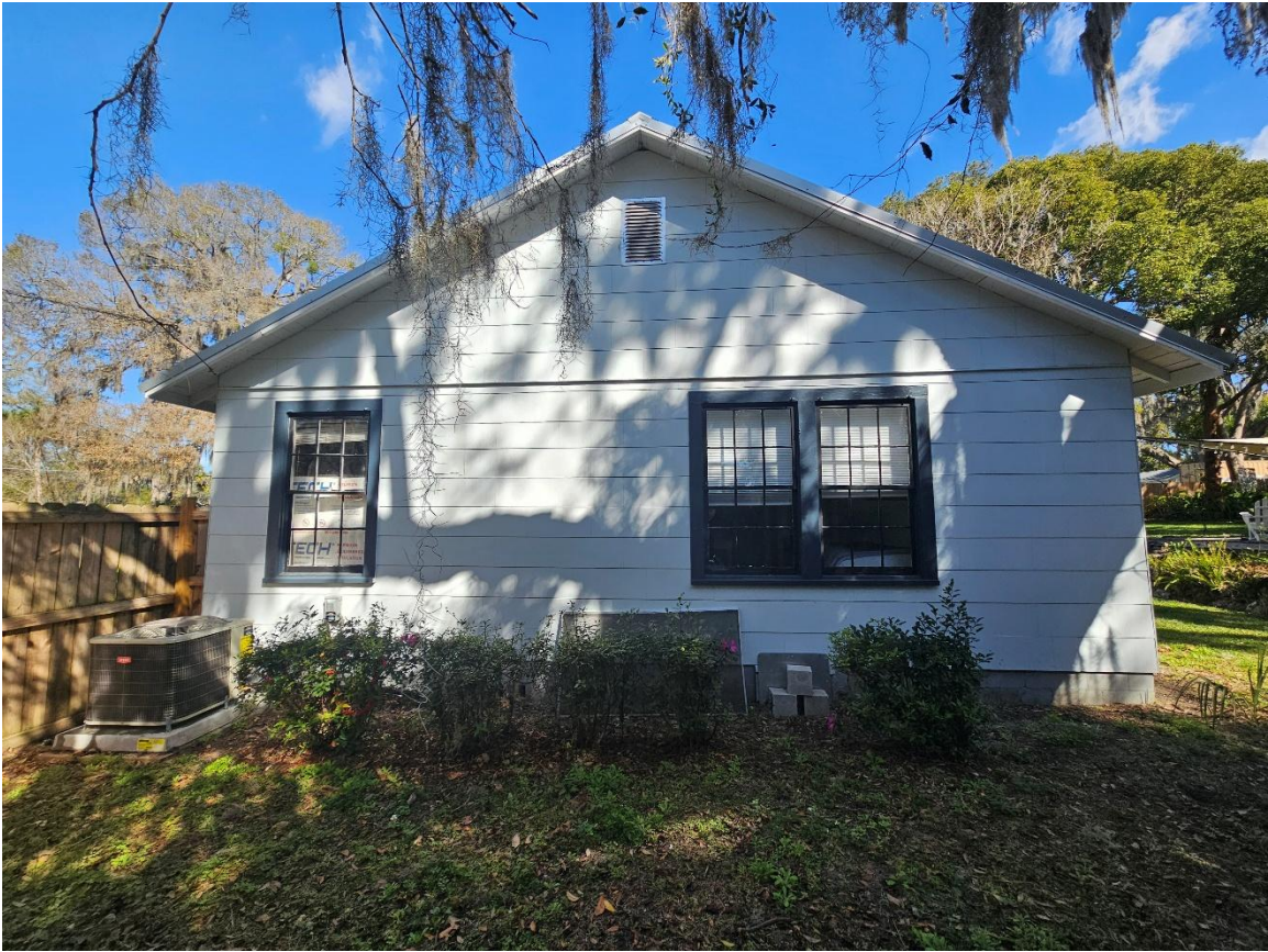
Image 3 – From the side of the property facing North.
