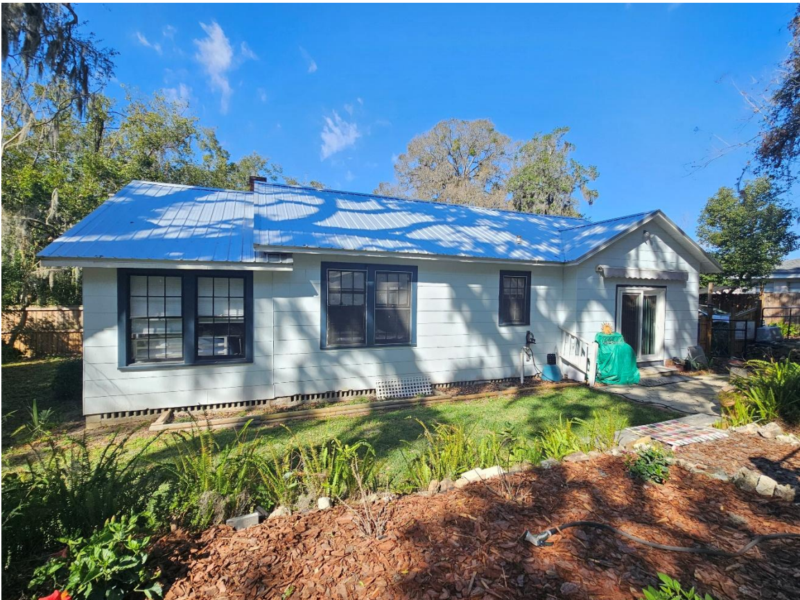
Image 4 – From the back of the property facing West.
