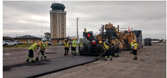
Taxiway “A” Construction
