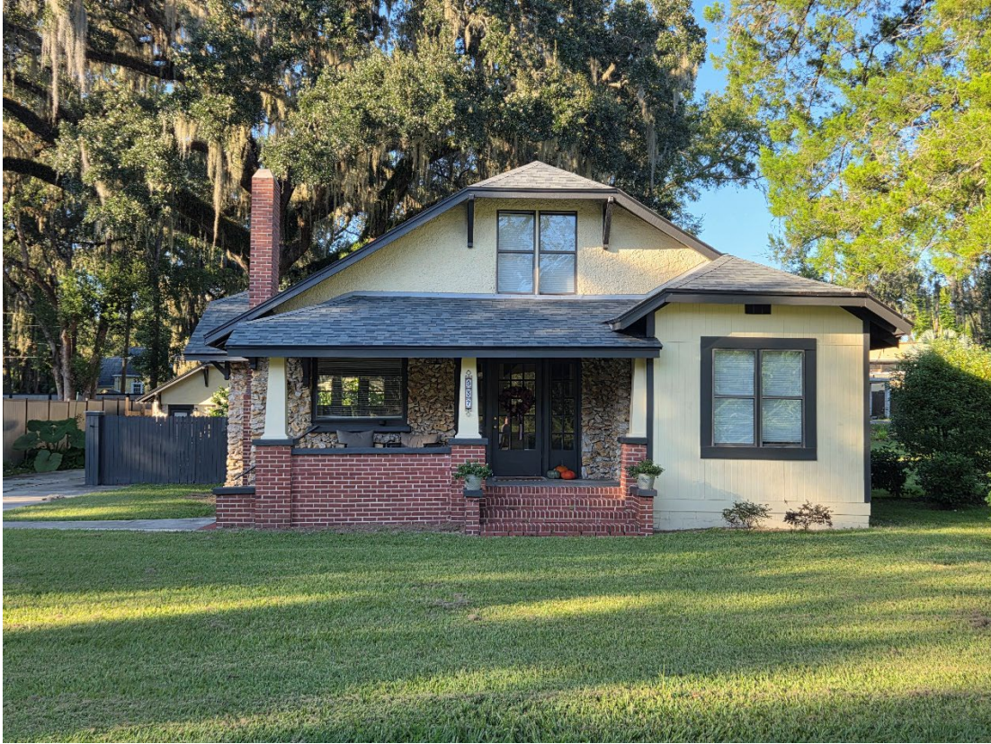
937 NE 3 rd St. Before Photos
