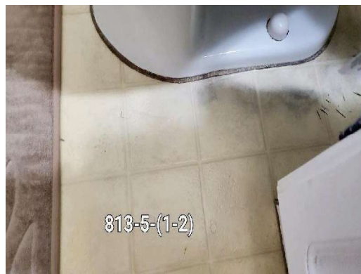
813-5 Rolled Flooring/White, Adhesive/Yellow Typical Interior Bathrooms
