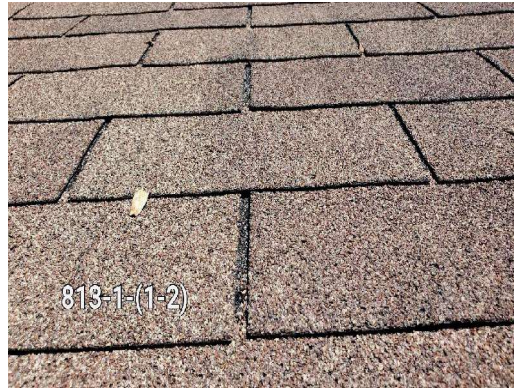
813-1 Asphalt Shingle/Black, Tar/Black Typical Exterior Roof
