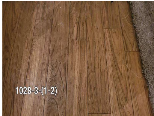
1028-3 Rolled Flooring/Brown, Adhesive/Yellow Typical Interior Floors
